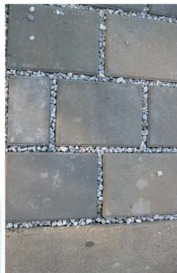
A property owner can reduce their SPF bill by installing stormwater management features on their property such as vegetated roofs, rain barrels, and permeable pavers.
