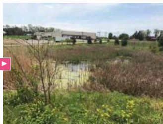
Constructed wetland at Dansko distribution warehouse in Penn Township, PA.
