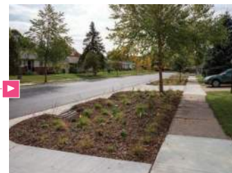
Tree trenches in Hoyer Heights, Minneapolis. (Photo credit- "Hoyer Heights Tree Trenches" by Mississippi WMO is licensed under CC BY-NC 2.0).
