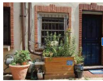
Residential downspout planter installed through the Philadelphia Water Department's Rain Check program. (Photo credit- "Downspout Planter" by Home Science is licensed under CC BY-SA 2.0).
