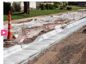
Construction of tree trench in Hoyer Heights, Minneapolis. (Photo credit- "Hoyer Heights Tree Trenches" by Mississippi WMO is licensed under CC BY-NC 2.0).
