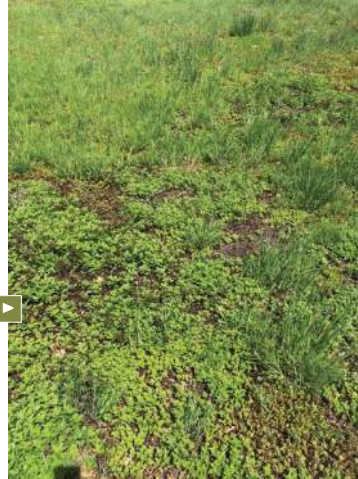
Typical green roof vegetation.
