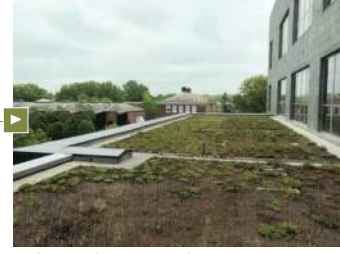
Green roof at University of Delaware, Newark, DE.
