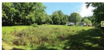
Residential bioretention basin in Westtown Township, PA.
