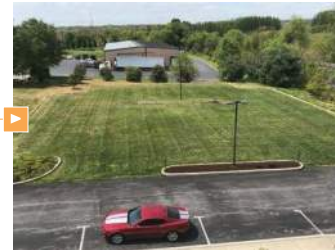
Pervious overflow grassed parking area at Dansko Company store and outlet, Penn Township, PA.
