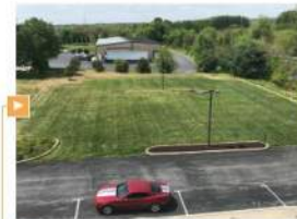
Pervious overflow grassed parking area at Dansko Company store and outlet, Penn Township, PA.
