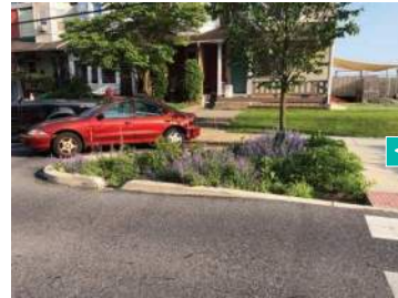
Crosswalk with stormwater bump-out in Lancaster City, PA.
