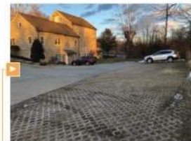
Pervious paver parking spaces at Chadds Ford, Chadds Ford Township, PA.
