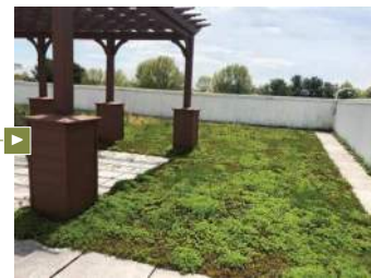
Green roof with pavilion and patio area at Dansko Company store and outlet, Penn Township, PA.
