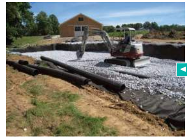
Installation of an underground infiltration system in Coatesville, PA.
