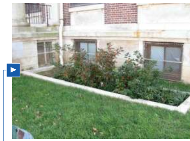
Large in ground downspout planter. (Photo credit- "Flow-Through Planters" by Michael Feagans is licensed under CC BY-NC-SA 2.0).
