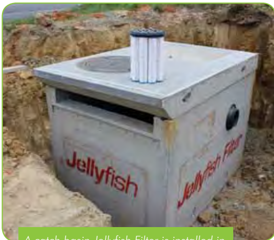
A catch basin Jellyfish Filter is installed in a commercial development in Virginia.
