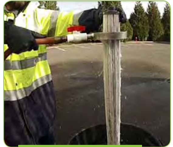
The Jellyfish Filter cartridge is light and easy to clean.
