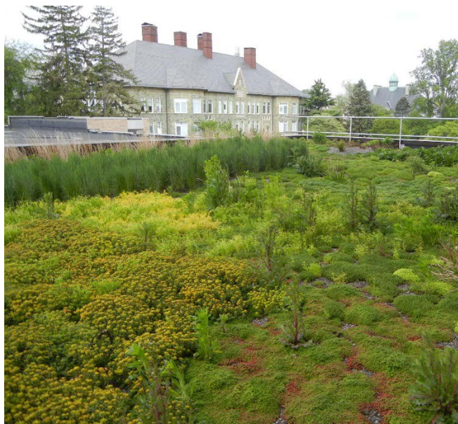
Green roof at West Chester University
