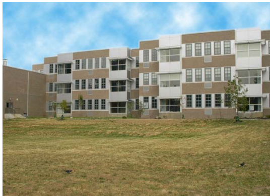
The Vegetated Infiltration Basin beneath this playfield manages rooftop runoff from the adjacent school building, Philadelphia, PA
