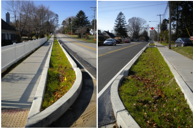
Vegetated curb extensions in Berwyn, PA Source: CH2M HILL
