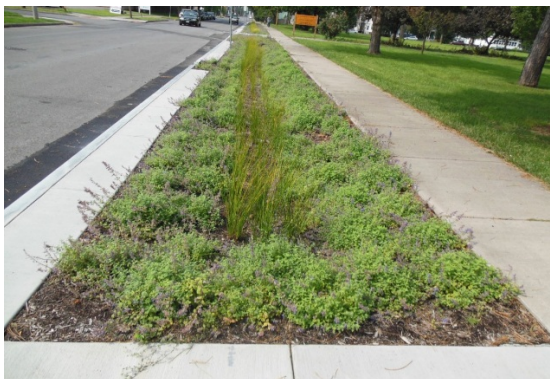
Right-of-way bioretention planting in Syracuse, NY
