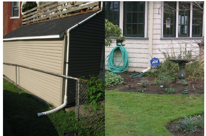
Residential downspout disconnect in Lancaster, PA and Portland, OR
